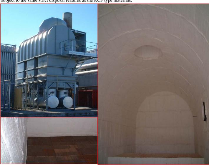
The lining was constructed from 1260c rated fibre materials Cerablanket 1260c, the modular lining was manufactured to a nominal density of 175kg/m3. Anchorage was 316 S/S studwelded
